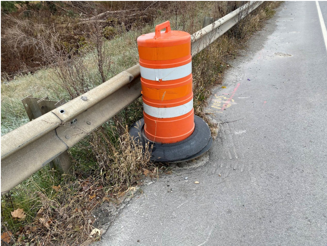
Depression along North Side with Barrel (Inspection photo 2021)
