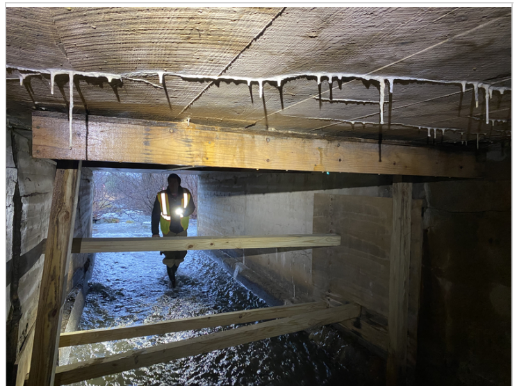
Timber Blocking to prevent further Spalling / Settlement in Roadway Near Upstream End / Below Approach Rail
