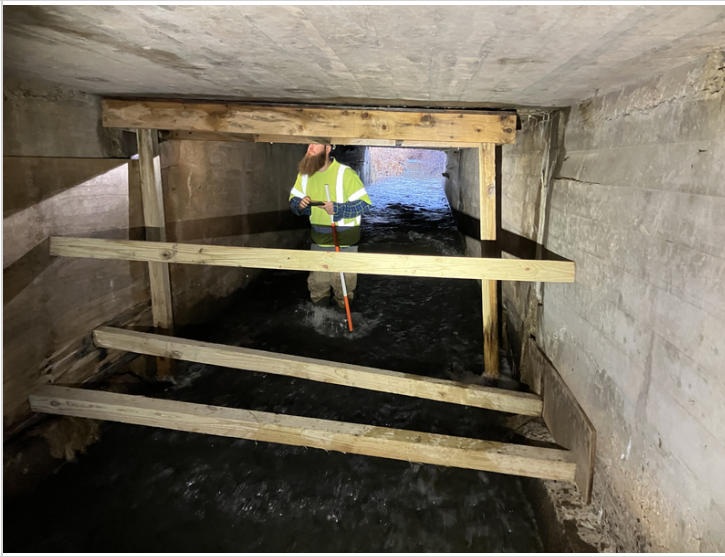
Timber Supports between Midspan and upstream End
