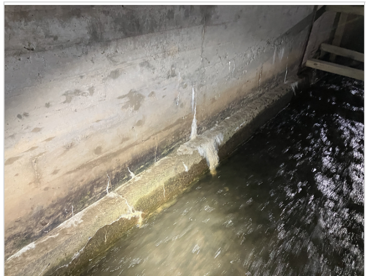
Efflorescence on Eastern Side of Culvert near Upstream End
