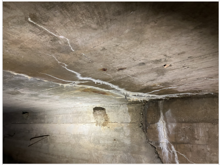
Cracking and Efflorescence and sagging along western side and top of culvert near downstream end
