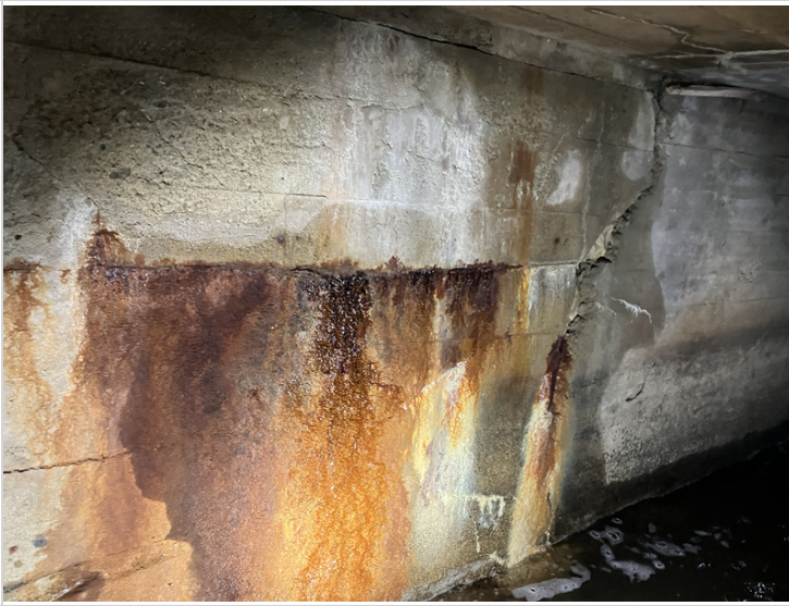
Cracking, Efflorescence and Rust staining on Eastern Side of Culvert near Midspan
