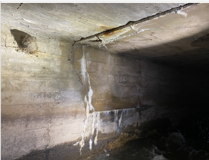
Displacement in Box with Heavy Saturation, Rust Staining and Efflorescence at Widening/Lengthening Joint Downstream
