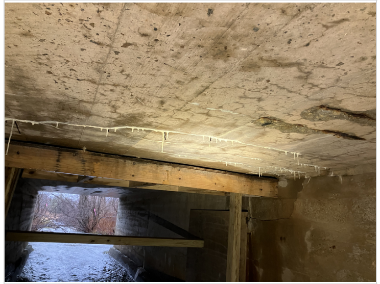
Cracking and Efflorescence on downstream Side of Timber supports
