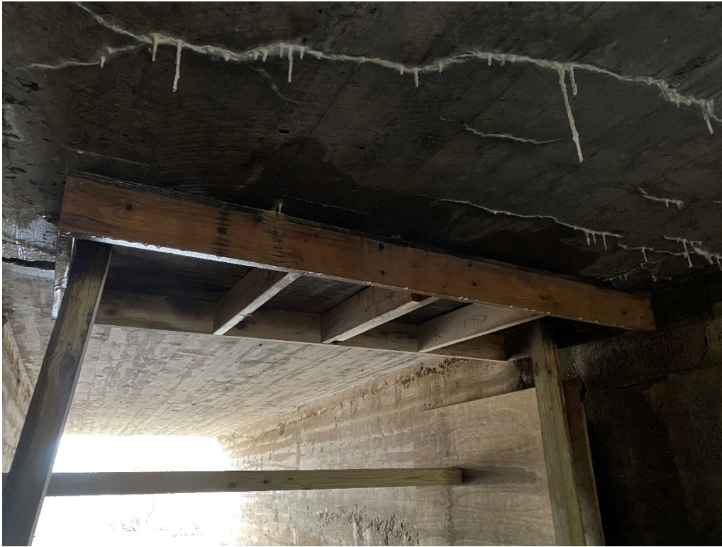
Timber bunker below Upstream Spall (Inspection photo 2021)
