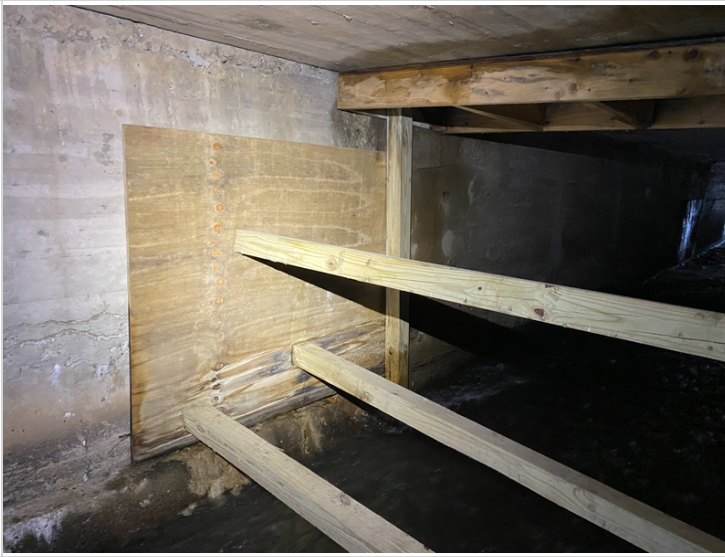
Timber Blocking to prevent further Spalling / Settlement in Roadway Near Upstream End / Below Approach Rail
