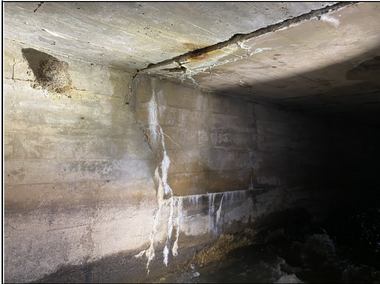
Displacement in Box with Heavy Saturation, Rust
