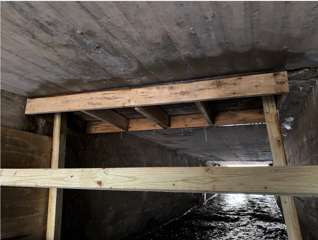
Timber Bunker (Inspection photo 2021)
