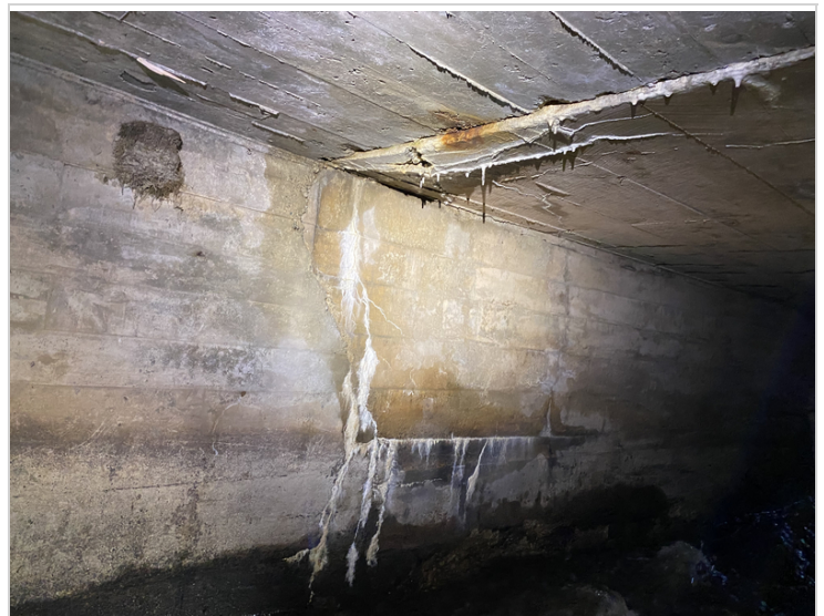
Displacement in Box with Heavy Saturation, Rust Staining and Efflorescence at Widening/Lengthening Joint Downstream
