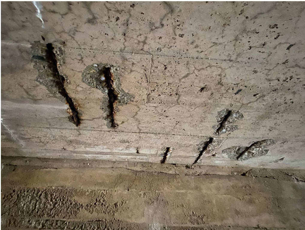
Box Soffit Shallow Rebar below Roadway (Inspection photo 2021)
