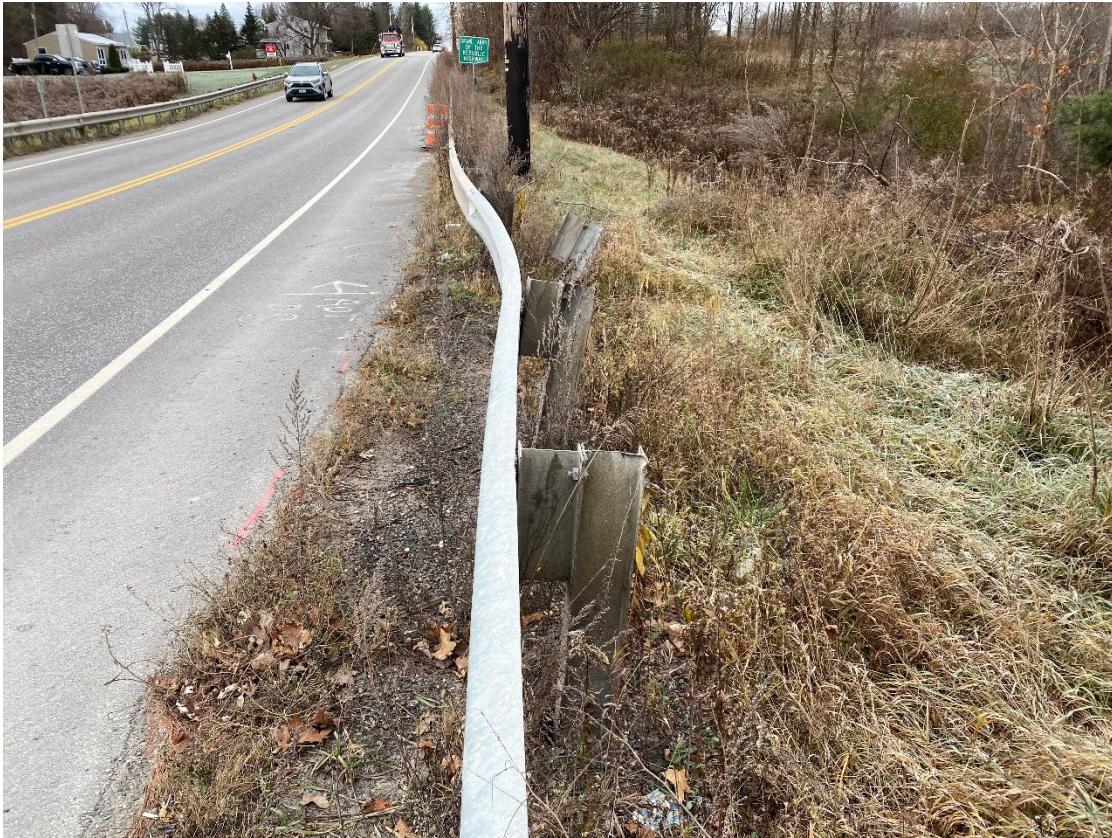
Impact Damage Northern Side Rail (Inspection photo 2021)
