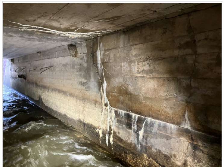
Cracking and Efflorescence on Western Side of Culvert near Midspan
